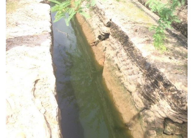
Canal linking the catchments
