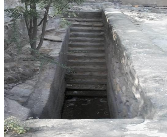
Water conservation and ground water recharge
